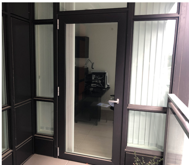
Figure 9 – Example of an aluminum frame swing door
