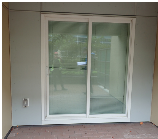
Figure 10 – Example of a vinyl frame sliding door
