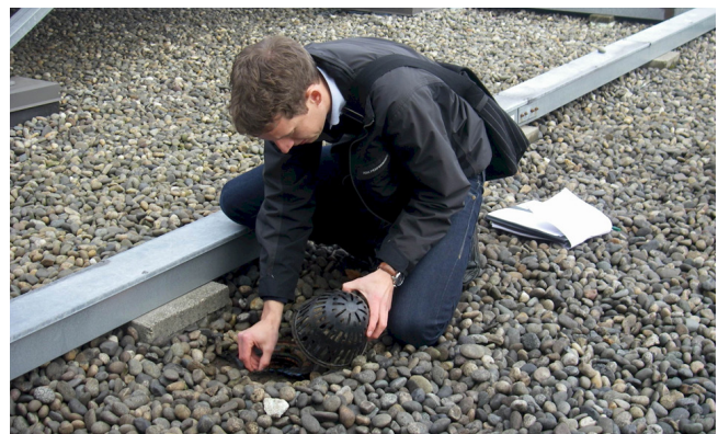
Roof drain cleaning
