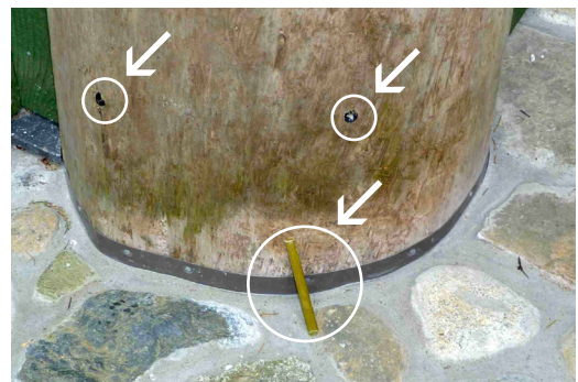
Installation of boron rods at base of post will provide greater resistance to decay. Boron rod shown leaning against base of post and locations where installed are highlighted by white arrows.
