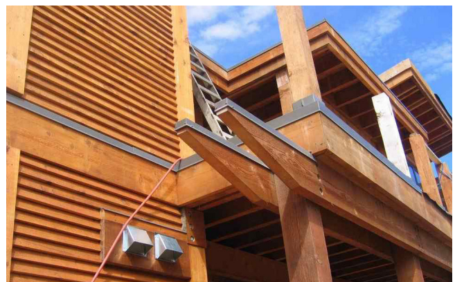
Metal cap flashing on exposed beam ends prevents water from collecting on the upper horizontal surfaces.
