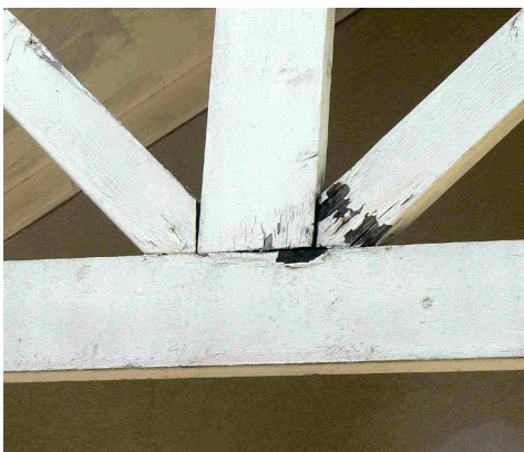
Open joints collect water and lead to deteriorated beams and columns at the connection.
