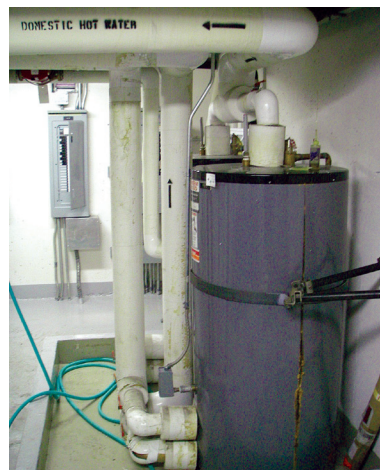
Central domestic hot water system
