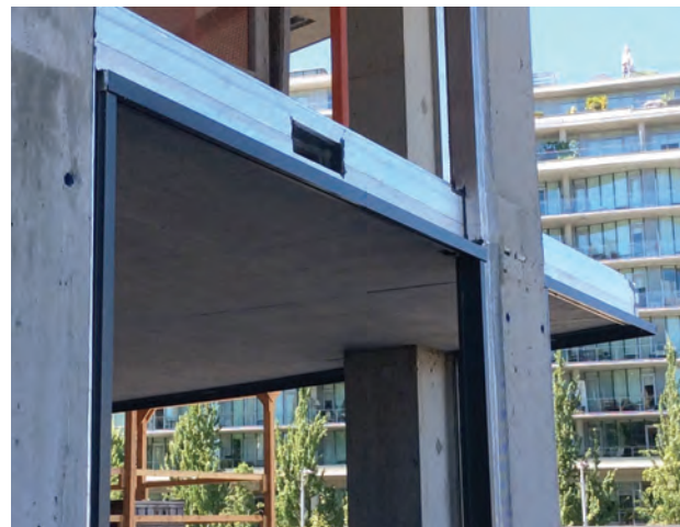
Waterproofing at the edge of the floor at the by-pass panel area
