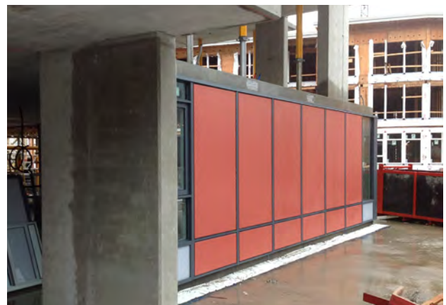
Metal spandrel panels
