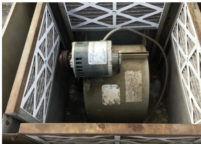
Figure 8: Inside an unheated MUA.
