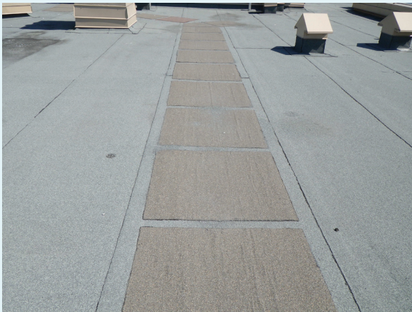
Figure 5: Sacrificial layer of waterproof membrane leading from the roof hatch to the MUA.
