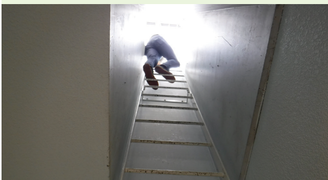
Figure 6: Roof access via hatch.
