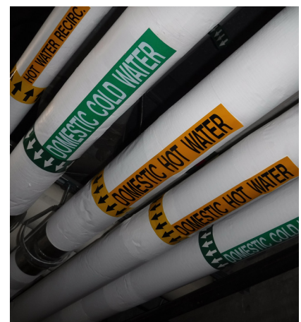
Example of domestic cold water and hot water piping wrapped in insulation
