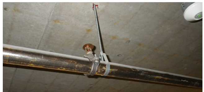
Example of a pipe mounted sprinkler head in a dry fire suppression system in the garage of a multi-unit residential building
