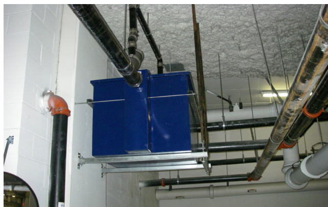
Example of a multichambered flow through grease trap suspended from the structure above
