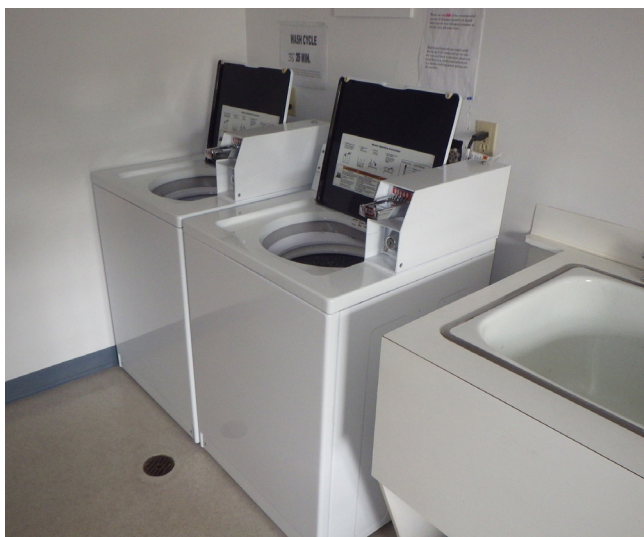
Example of a communal laundry room with a built-in drain in case of washing machine back-up, overflow or leaks
