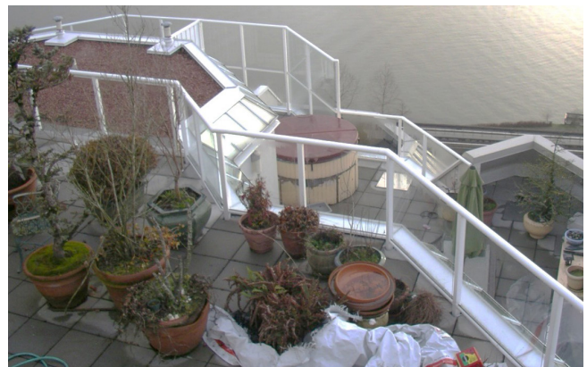
Example of live loads on decks.
