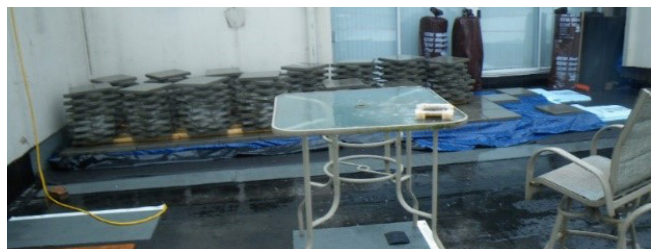
Stacked concrete pavers during membrane repair work
